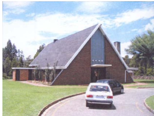
Figure 046: Photograph of entrance to Pretoria Crematorium chapel.
