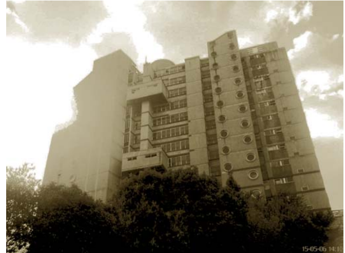
Figure 007: Photograph of the 15 storey Drie Lelies South Block
