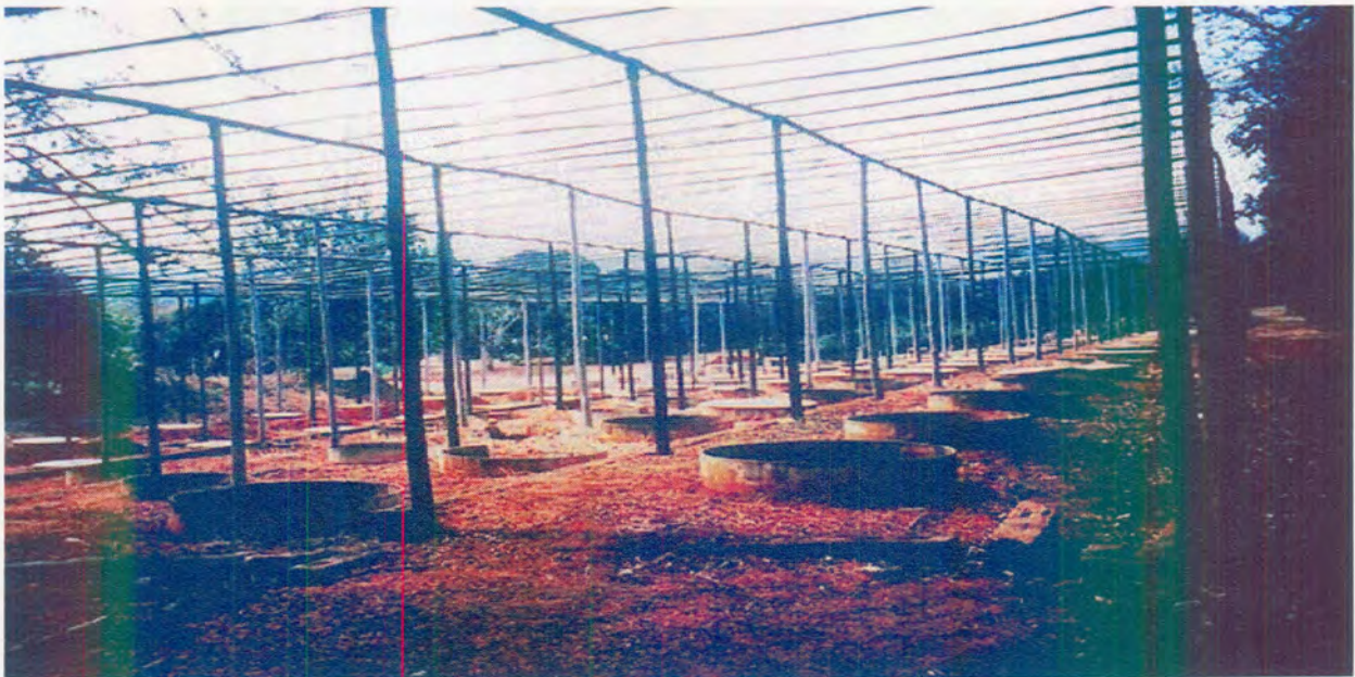
Figure 3.2 Old shade cloth structure during the process of renovation.
