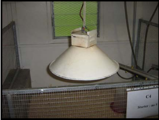
Figure 5.3. Heater hanging from the roof
