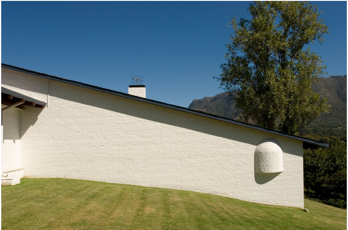
Figure 6.22. East edge of living room at House Keurbos (1951) (Photo courtesy of Leon Krige photographer, 2010).
