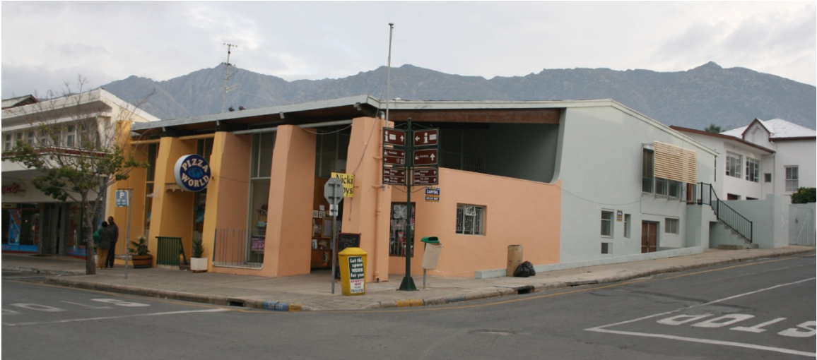
Figure 6.28. The Montagu branch of Volkskas as it existed in 2008. The street presence and corner treatment are still strong features while some of the interiors have survived in the new commercial arrangement (Author, 2008).
