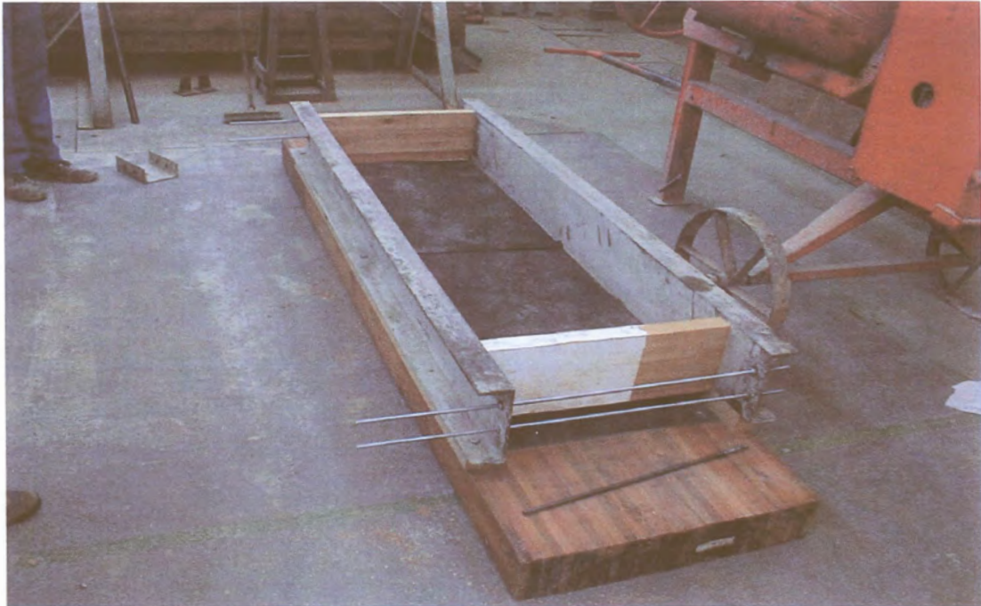
Photo G.1: Shuttering
