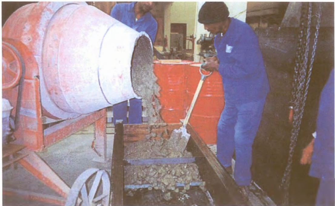
Photo G.2: Casting concrete – crack inducer and crack former in place in mould
