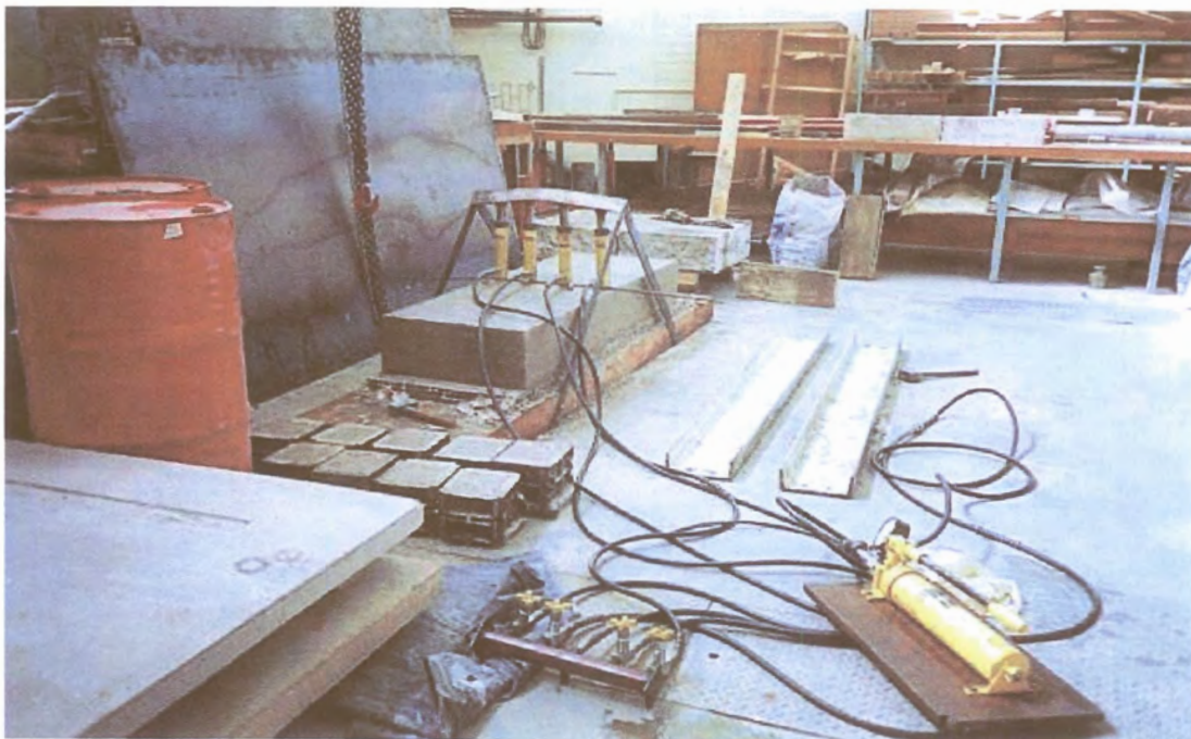
Photo G.4: Forming crack within 24 hours after casting beam
