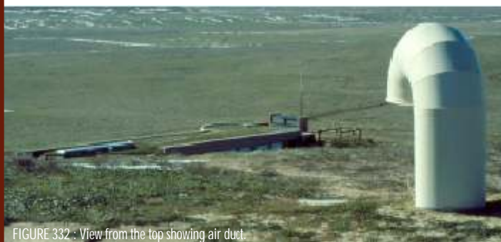
FIGURE 332: View from the top showing air duct.
