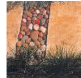
FIGURE 301: Pebbles and concrete blocks.
