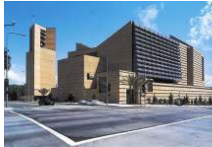
FIGURE 163: Exterior view from Grand Avenue
