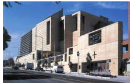
FIGURE 165: Exterior view Temple Street.
