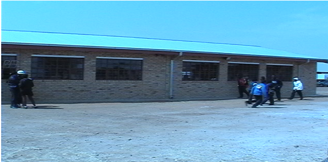
Self produced photograph (28/03/2003) 3 (e): shows the new additional administration block built from the infrastructure capital project.
