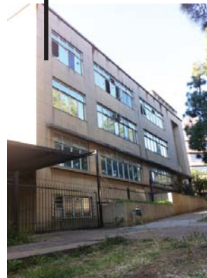
Fig.256: Clear distinction of different phases of the Agrivaal building due to material use. [Source: author 2011]
