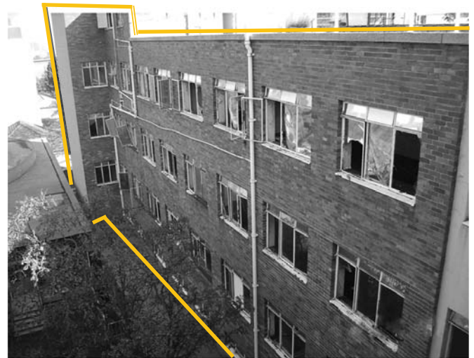
Fig.260:Phase 3 addition of the Agrivaal Building, 1953. [Source: author 2011]
