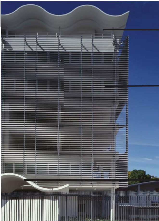
Fig.294: louvers, fencing, roof. [Source: www.bdp.com/Projects/By-Name/P-Z/Umoja-House/]
