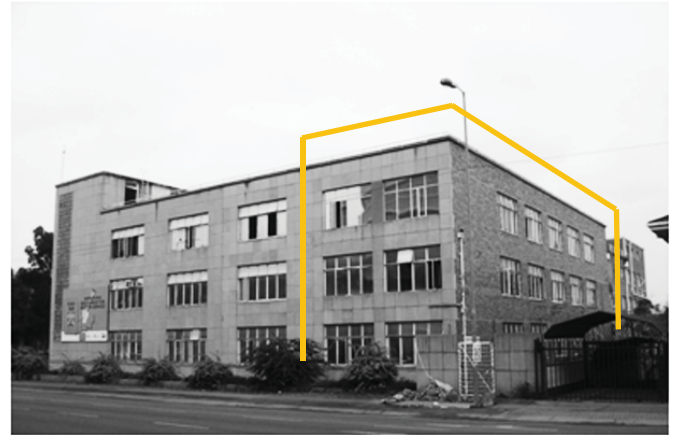
Fig.259:Phase 2 addition of the Agrivaal Building, 1946. [Source: author 2011]
