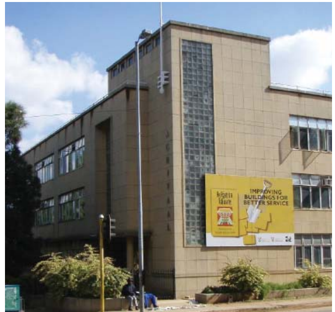
Fig.263: Glass blocks used to accentuate the corner articulation of the Agrivaal Building [Source: author 2011]
