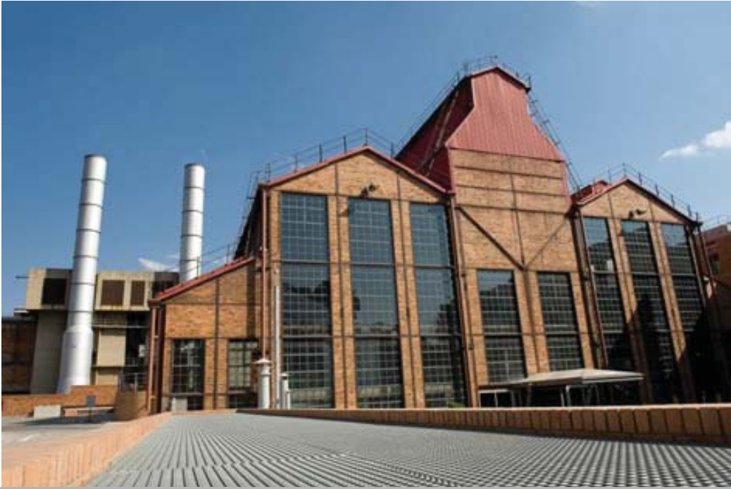
Fig.296: Turbine Hall [Sourced: www.conference-venues.co.za/gjhb_forumturbine.htm ]
