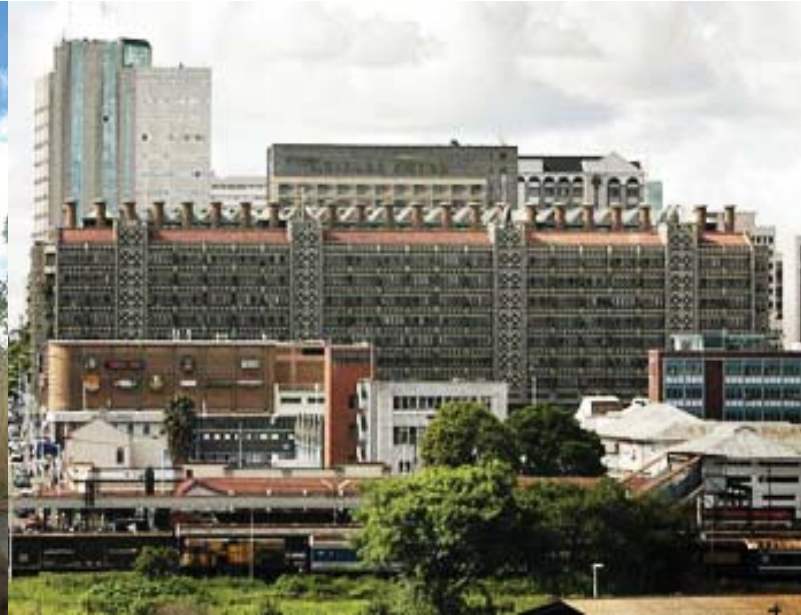
Fig.221:Eastgate Centre elevation, with chimney vents allowing air to escape the building. [Source: www.nubianarchitects.wordpress.com/2010/08/16/termite-and-temperature-control-from-zimbabwe/ , accessed 2 October 2011]
