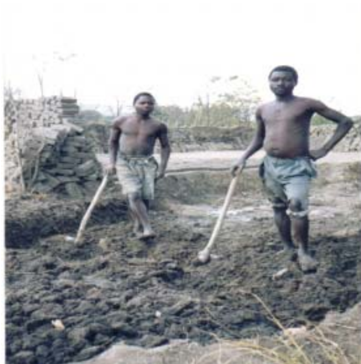
Figure 4: Moulding bricks from Dambo soils for construction purposes.
