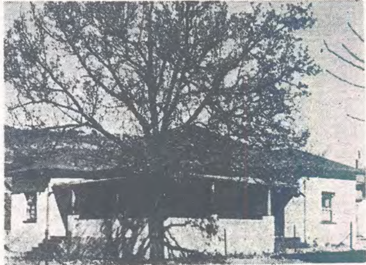
NOW — This house now stands on what is believed to be the site of Jess' Cottage. (Photos by C. A. van Tilburg.)
