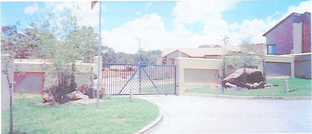
Figure 5.2 - The secured property development
