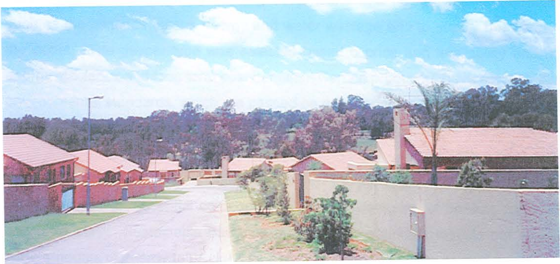
Figure 5.15 - The development with tarred road and central lighting, grassed frontage and new planting. The electrical supply and telephone exchange box are visible
