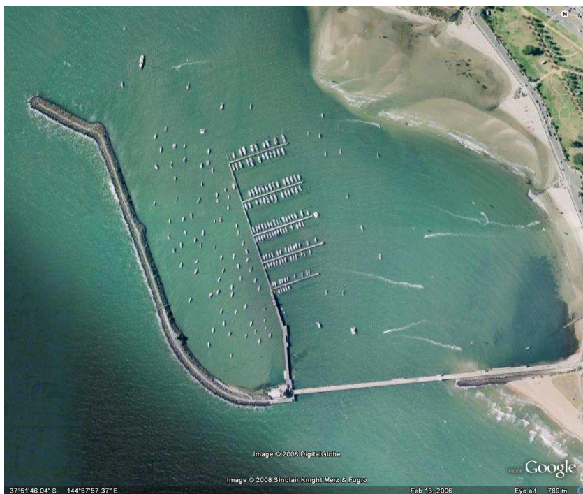
Figure 2-10: Satellite image of the St Kilda pier and breakwater (taken from Google Earth™).
