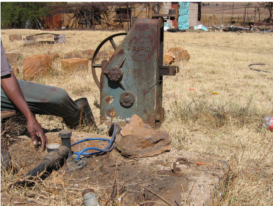
Figure 4.8: Sisonke farming project – borehole
