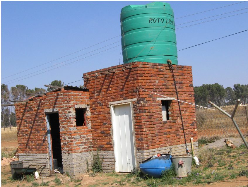
Figure 4.9: Soko Wilfred's farming project – pump house with tank
