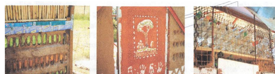
Fig.115: In-fill panels developed at the 'Green Wall project (Brewis, 2003:17 cited in Araujo, 2004:112).
