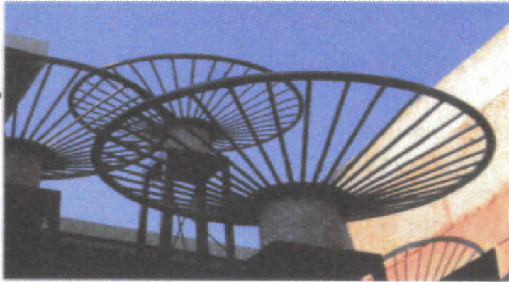
Fig.45: Steel basket tops (SA Digest, 2001:161).
