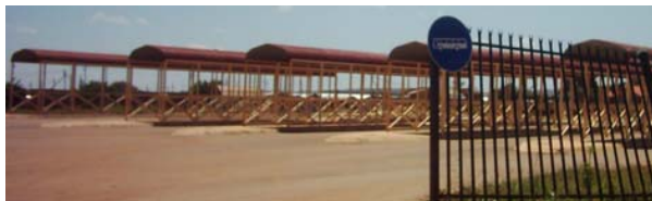
Fig.26: Exit from Bus station on Moretlwa street (author).
