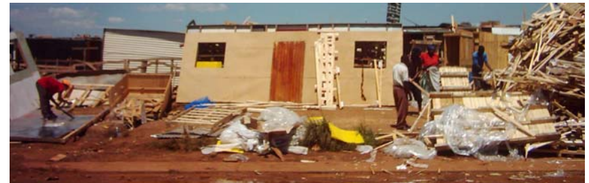
Fig.30: Shack panels made of steel sheets and timber assembled and made of site (author).
