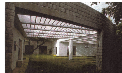
Fig.52: a view of one of the private green places between the wall and the work area (Steel, 1998:48).
