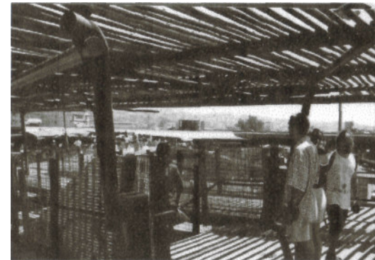
Fig.46: The combination of steel construction and reed cladding reflects the influence of traditional African building techniques within modern day African context (KZNA Journal vol3 2001:31).
