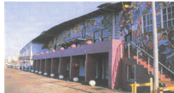
Fig.36: Façade of the BAT Centre with art, murals and bright colours (SA Digest, 1997:25).
