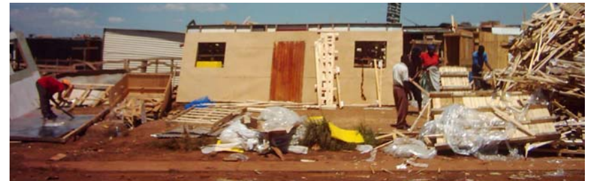
Fig.30: Shack panels made of steel sheets and timber assembled and made of site (author).
