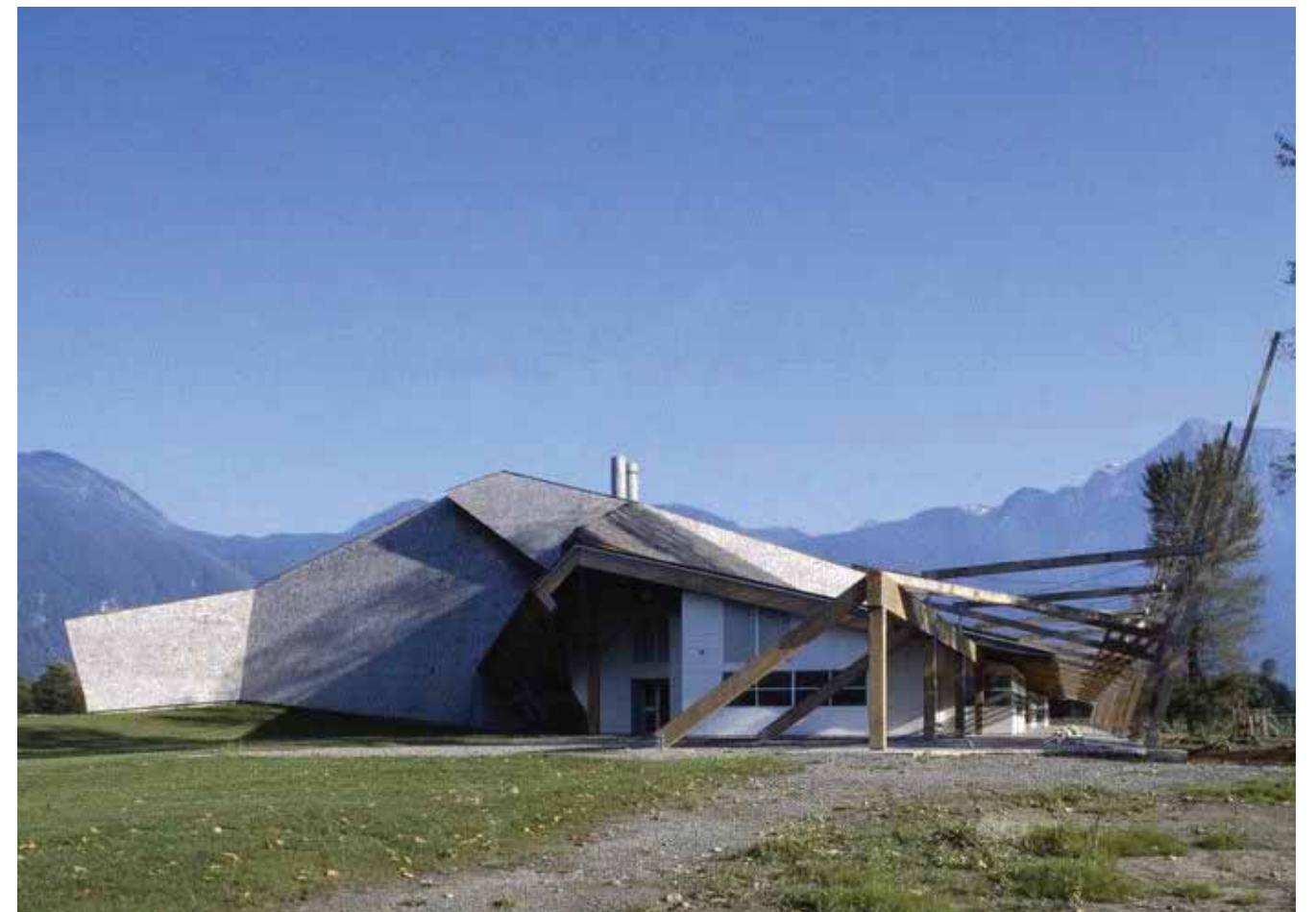
Figure - 6.4 - The building is organised around the porch with the bulk of the building situated on the northern side and connections to other community activities to the south.
