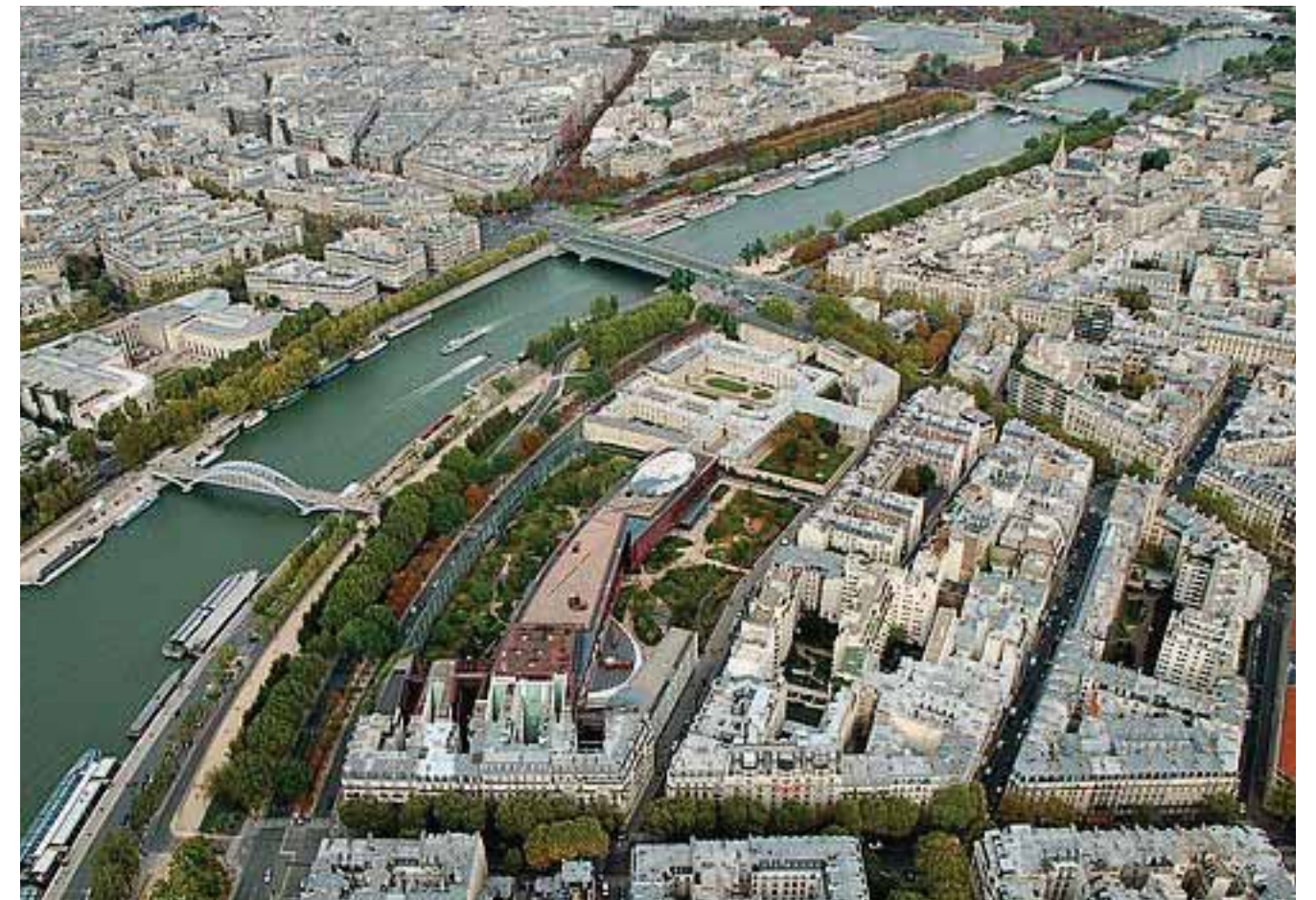
Figure - 6.21- Photograph from the Eiffel Tower depicting the greater context on the building.
