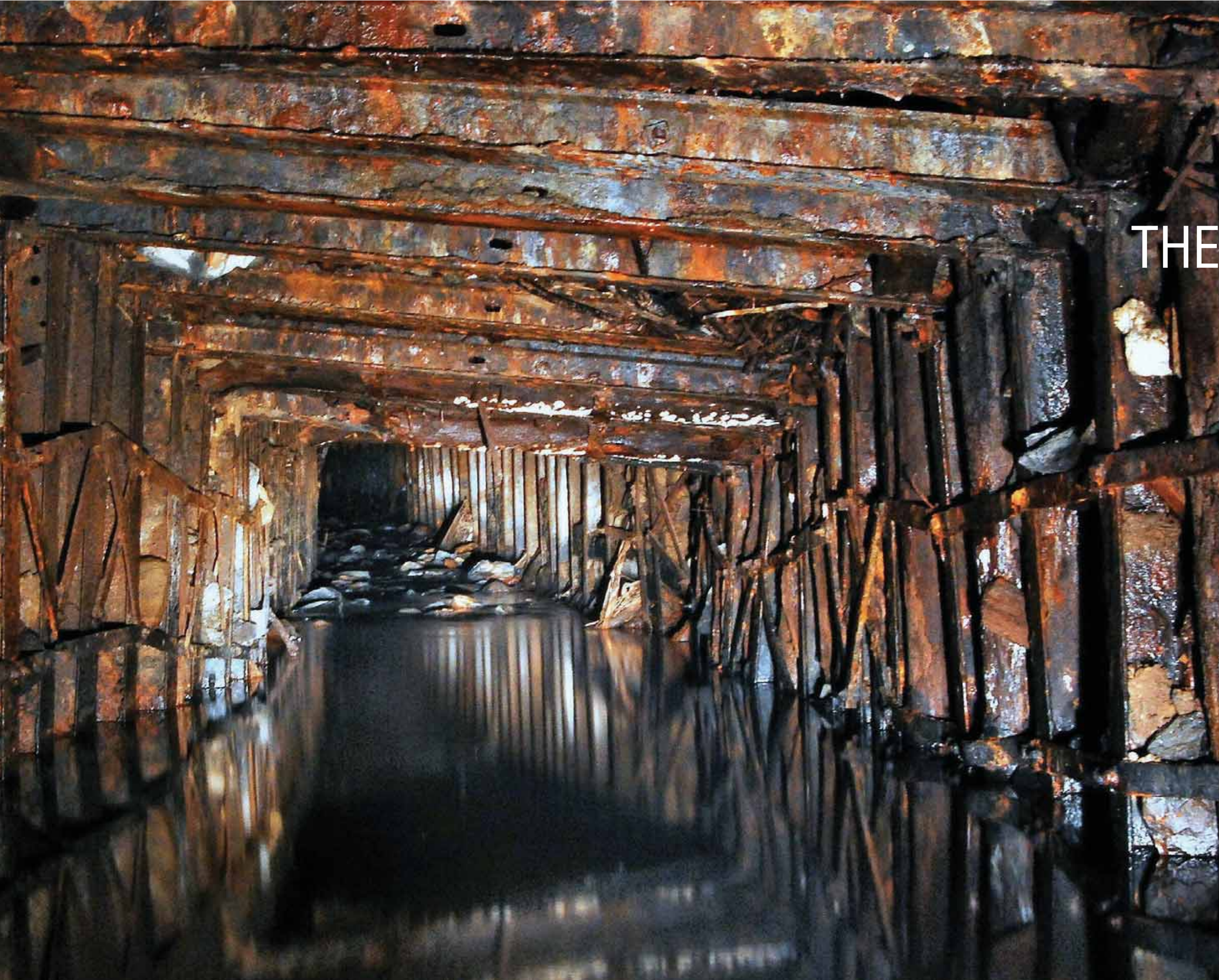
Fig - 3.1 This photograph is from Phil D's photographic col- lection of derelict indus- trial buildings. All photos Available on www.Flickr.com
