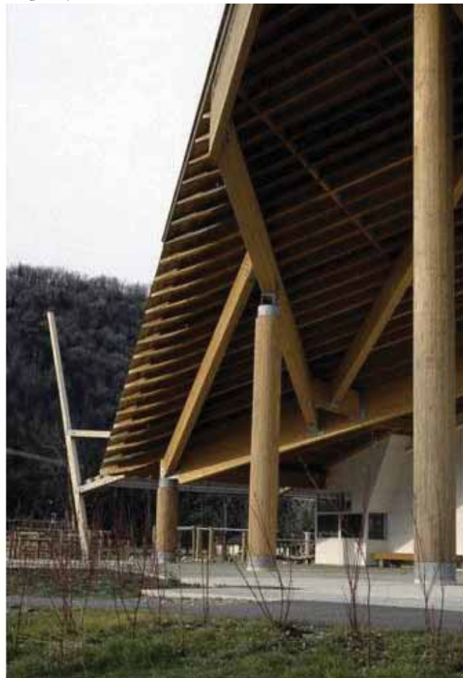
Figure - 6.2 - The heavy engineered timber post and beam construction.
