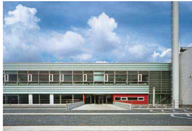
Figure - 6.10 - A completely different aesthetic was used compared to the typical industrial sheds.
