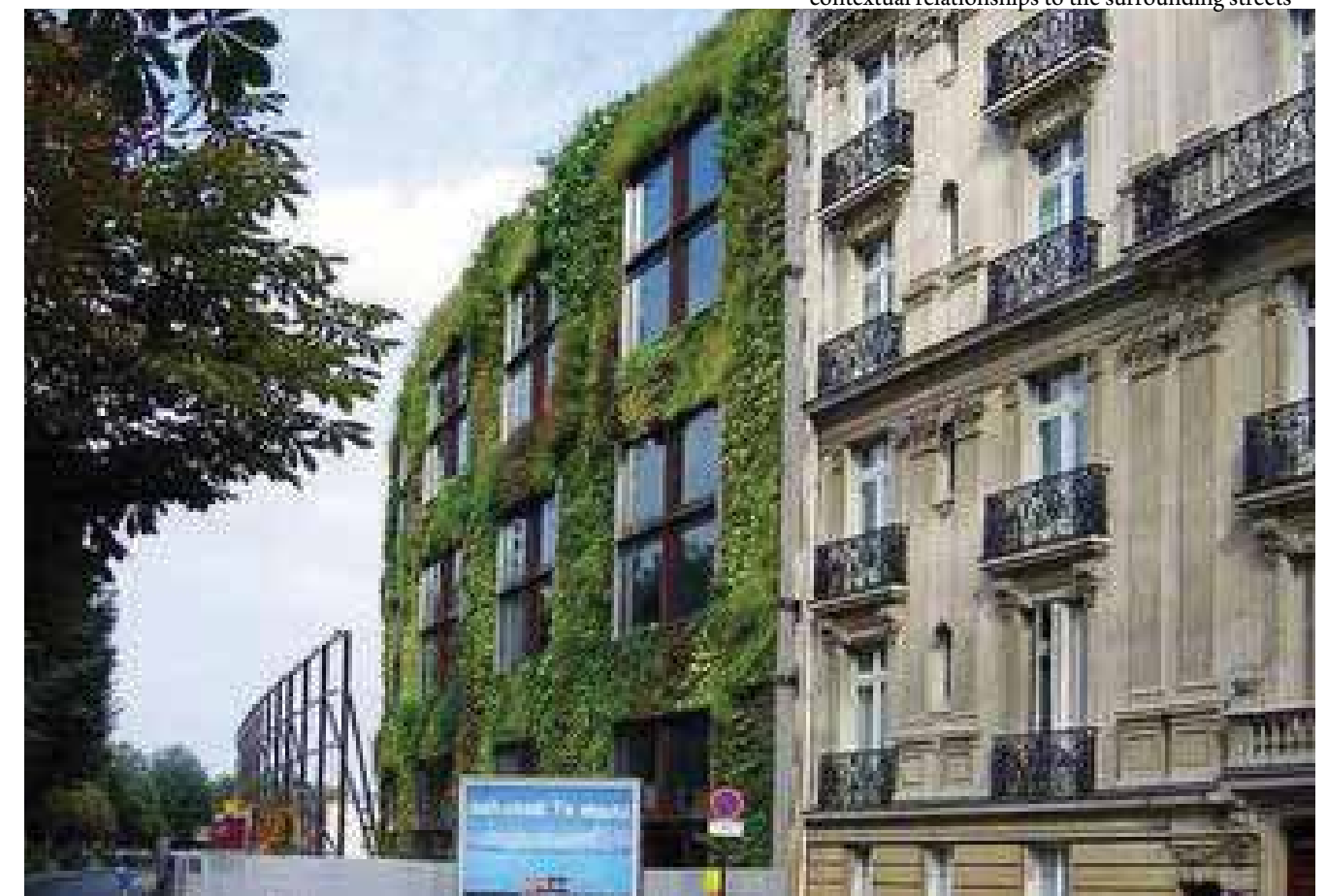
Figure - 6.26 - The existing building facade is continued, but the new is characterised by large windows and a wall which is completely planted.
