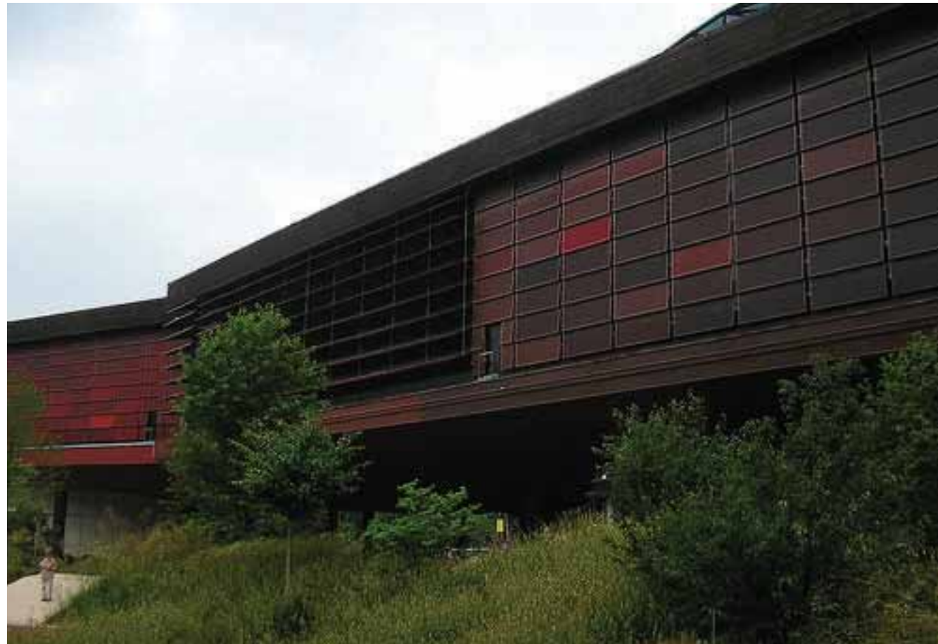
Figure - 6.23 (Below) - The envelope of the above ground exhibition space consists of a series of adjustable louvres to control the light inside the exhibition. The site is also heavily planted with trees, converting a Parisian garden into a forest with a museum hidden inside.
