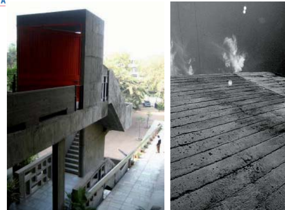
Figure 12.38 Textured off-shutter concrete of the Millowners Association Building, 1955, Le Corbusier
