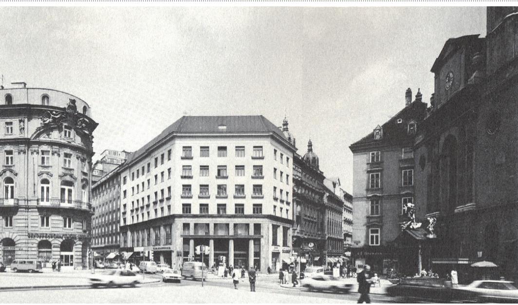
Figure 8.01 Goldman Salatsch House (centre), Vienna by Adolf Loos (1911)
