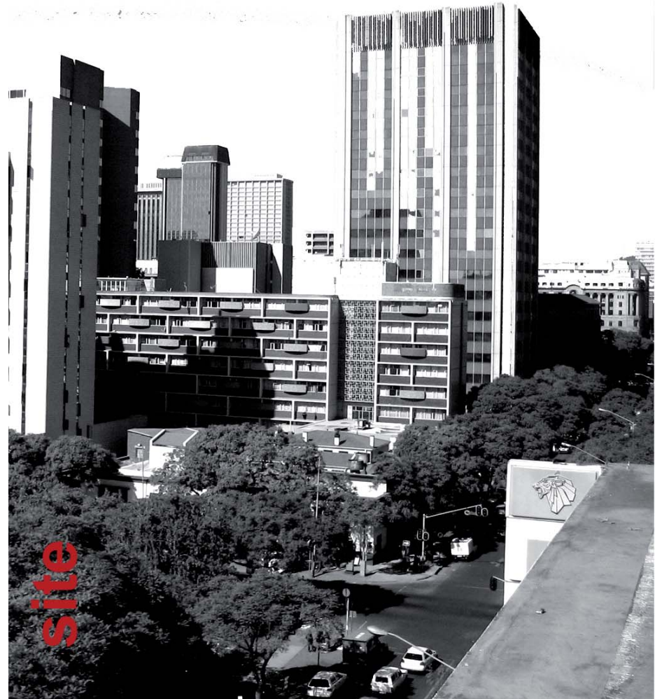
Figure 6.09 View south of threshold
