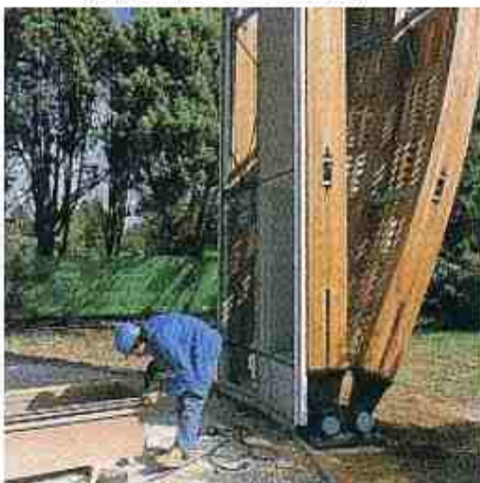
Fig.69 Traditional wooden cases made of laminated iroko an African wood braced with galvanized steel connectors (Architectural Review 1992:54)
