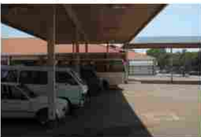
Fig.48 Vacant shops leads to dead space (Author, 2007).
