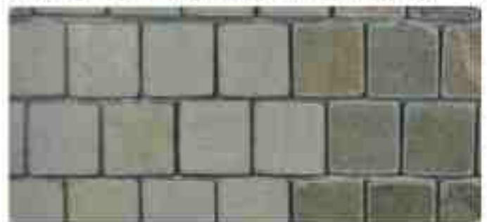
Fig.156 Floor Finish (Architecture SA 2007:3)
