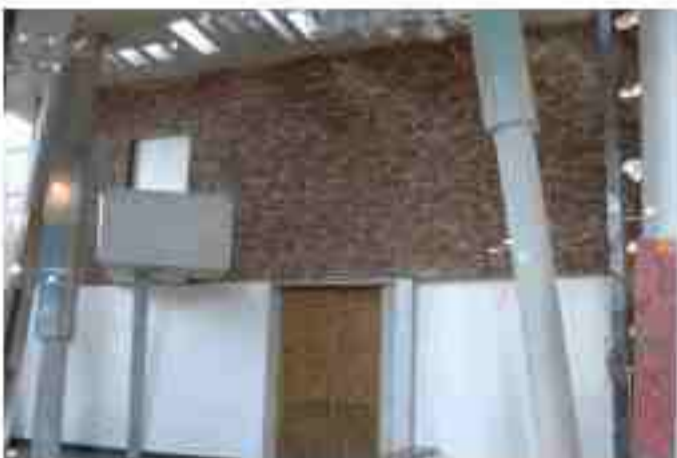
Fig.63 The colour of the finish on the new columns forms a continuity of the old building matching the old and new to read as one. Used face bricks has been adapted on the new walls to overcome the line of old and new structure (Author, 2007).
