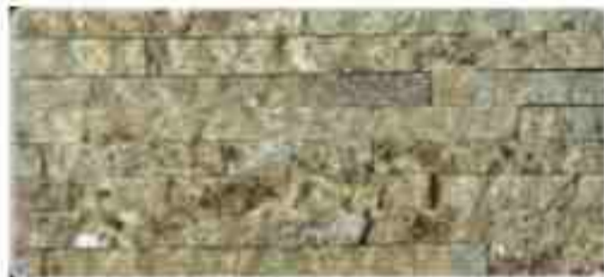
Fig.153 Wall Finish (Architecture SA 2007:3)
