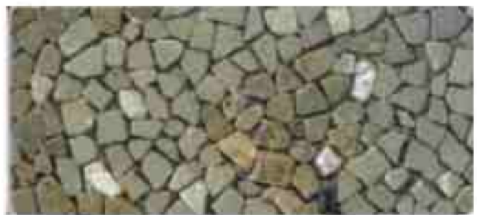
Fig.155 Floor Finish (Architecture SA 2007:3)
