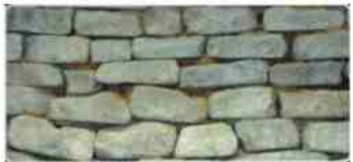
Fig.154 Wall Finish (Architecture SA 2007:3)
