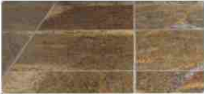
Fig.158 Floor Finish (Architecture SA, 2007:3)
