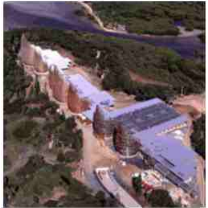
Fig.65 An aerial view of the Jean-Marie Tjibaou Cultural centre during construction (Architecture 1998:99)
