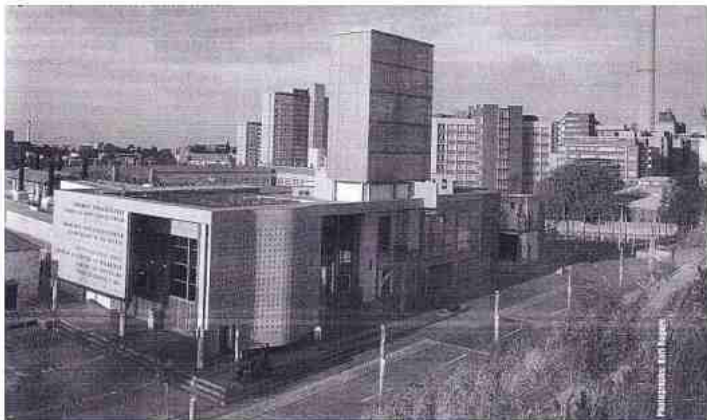
Fig.58 The Constitutional Court building (Leading Architecture 2004:81)
