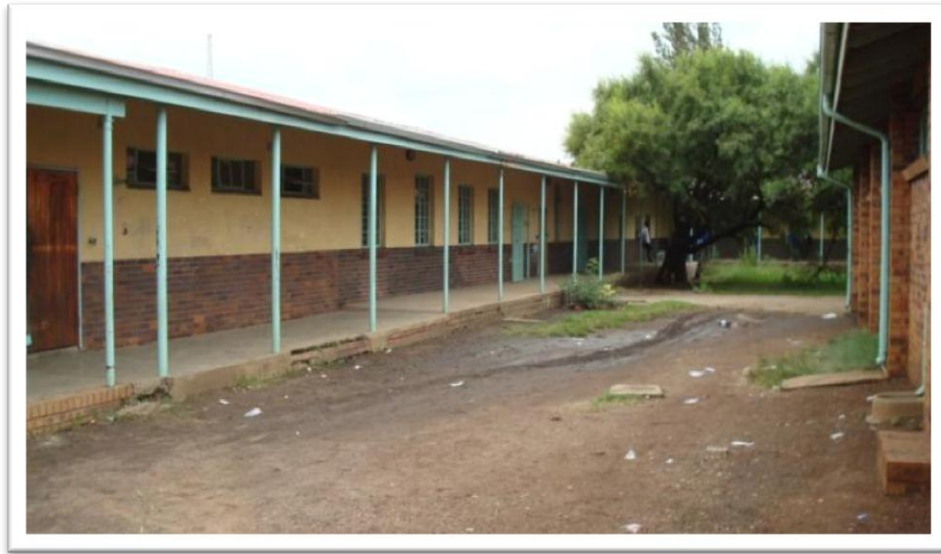
Figure 4.3: Classroom block at Mr Sogo's school
