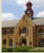
Old arts building 1911
