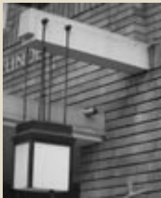
Detail of external lighting, Botany building 1940-59
