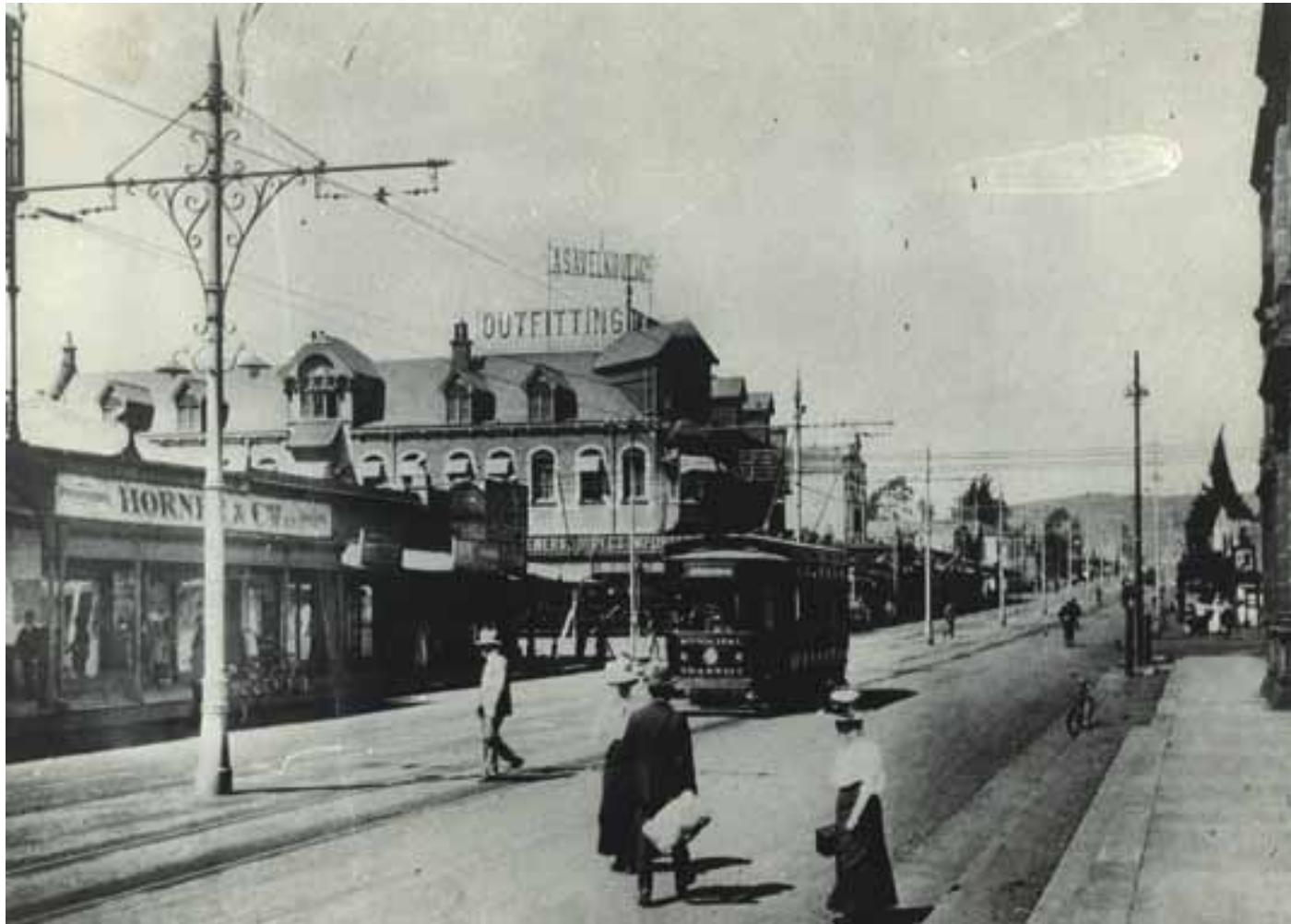
FIG. 4.2 View of tram line along Paul Kruger Street
