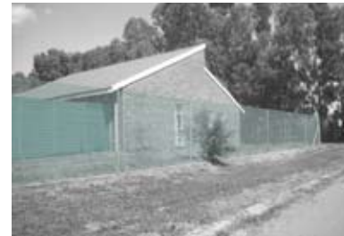
Figure 3.30. (far left) retaining wall as a boundary(Author 2009)
