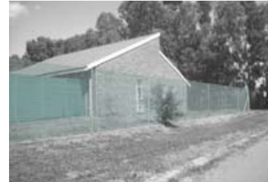
Figure 3.30. (far left) retaining wall as a boundary (Author 2009)
