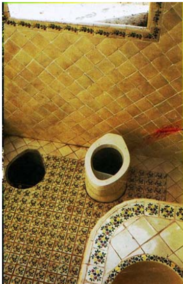
Figure 2.9: The Mexican version of the Vietnamese double-vault toilet, installed in the bathrooms of modern houses in the city of Cuernavaca. The toilets have movable urine-diversion pedestals. The processing chambers below the bathroom floor are accessible from outside the house (César Añorve, CITA, A.C., Mexico)
