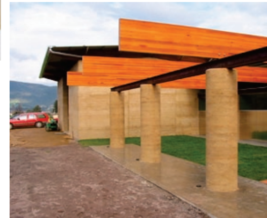
Fig185: Rammed earth wall joint
