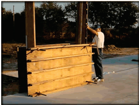
Fig191e: Wall going up
