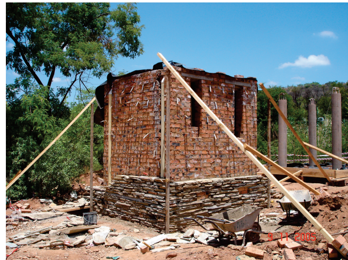
Fig170: Freedom Park features stone cladding which appears dry packed, but is fixed with steel ties to masonry structures
