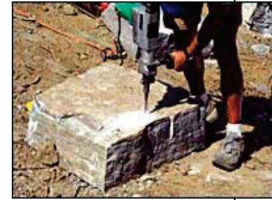
Fig163 - Fig 169: The process of building dry packed stone retainer walls requires specialised skills
