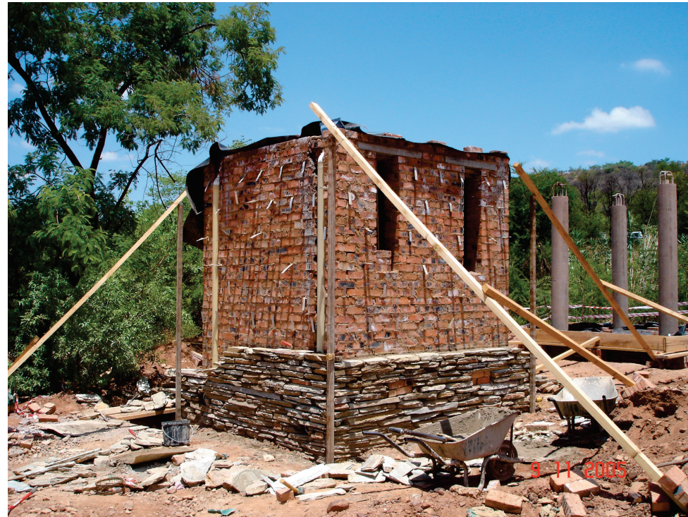
Fig68: Cladding is held onto the masonry wall with galvanised steel ties
