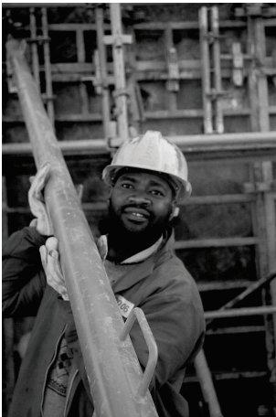
Fig67: Monumental scale casting of concrete
