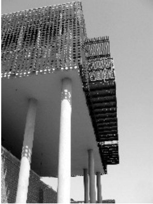
Fig. 5.20 The building protrudes over the original jail wall.
