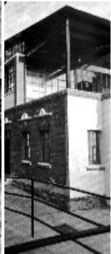
Fig. 5.7 The Drill Hall
