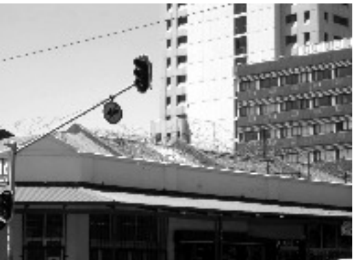
Fig.4.4 Safety is an issue, depicted by the barbed wire keeping potential thieves from entering via the roof
