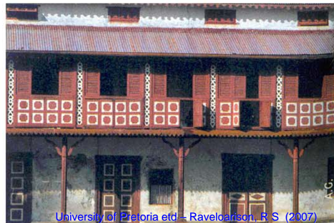
FIG. 18: A BUILDING FAÇADE DEMONSTRATING THE USE OF LOCAL MATERIALS - TIMBER, CORRUGATED STEEL ROOF SHEETING, AND MASONRY; USE OF MOTIFS - ABSTRACTED "ALDALO" OR MALAGASY TOTEM AND GEOMETRIC PATTERNS FOR THE OPENINGS; USE OF COLOURS - HERE DARK BROWN & WHITE PAINTS (SOURCE: GROUPEMENT INTERPROFESSIONNEL HOTELIER ET TOURISTIQUE DE NOSY BE. 2005: 8).
