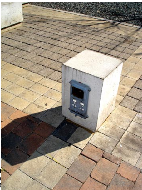
Fig. 3.13 Electrical points on the plaza (author, 2006)
