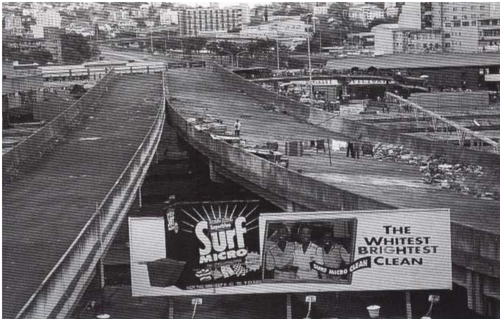
Fig. 3.1 Condition of bridge before herb traders started using it (Dobson, 2001)
