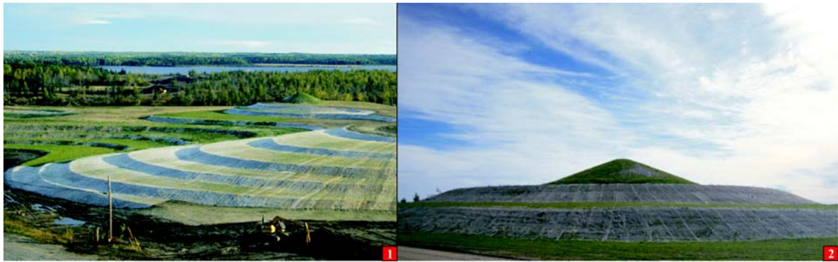
1 and 2 The McLeod High tailings impoundment was reshaped to create an environmentally stable sculptural landscape (photographs courtesy of Martha Swartz Partners).
