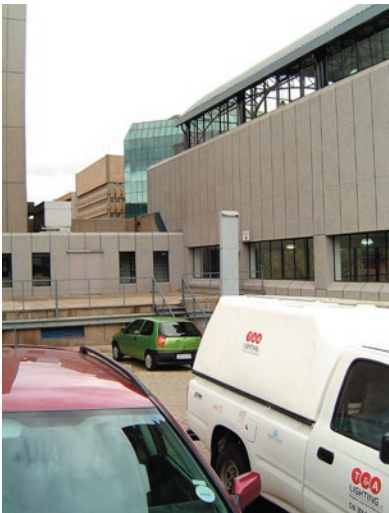
Fig 4.9: The eastern façade of the building also showing the link passage.
