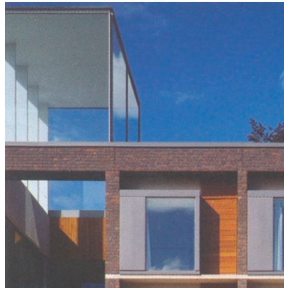
Fig 6.4: Fitzwilliam College Gatehouse and Auditorium _ Cambridge. Allies and Morrison.
