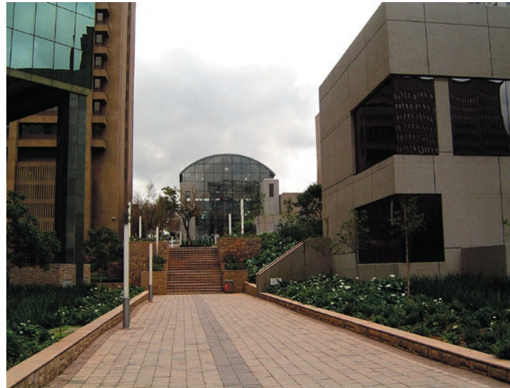
Fig 4.8: The pedestrian boulevard with the Johannesburg Civic Theatre to the right and the South African Ballet Theatre forming the focal point at the northern tip of the boulevard.
