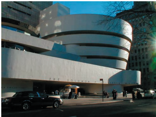
Fig 2.6: The Guggenheim Museum - New York City - the ‘spiral’ layout sends the user on a defined journey through the building.
