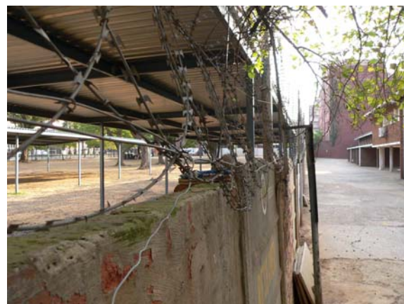
Fig 5.10h. St Alban's Cathedral's site
