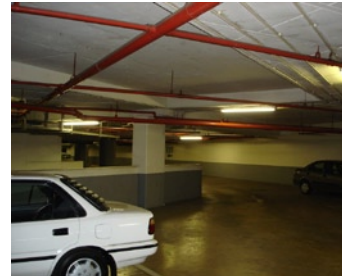
Fig. 5.10. Interior of the HSRC parking garage.
