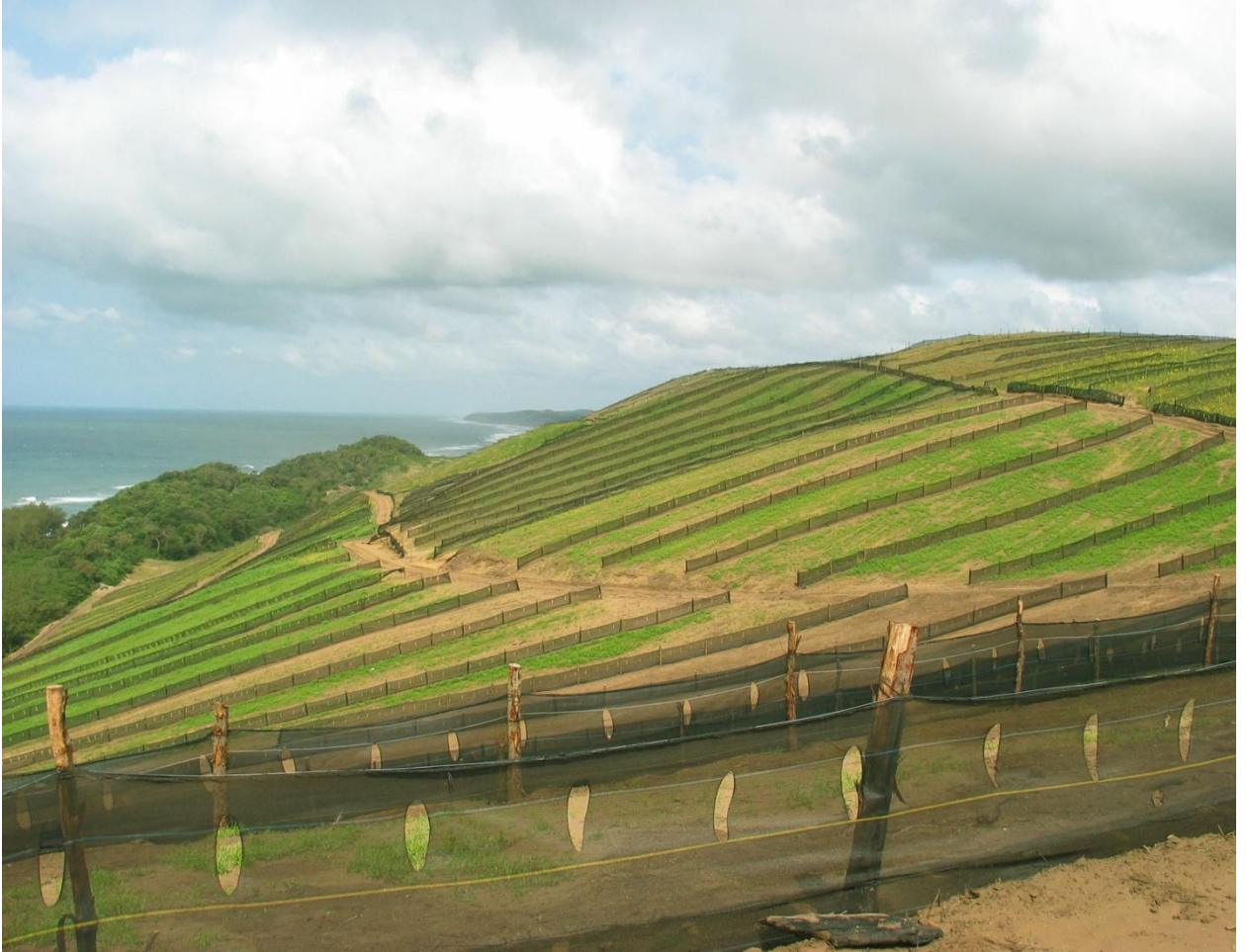
Plate 7-1. Post-mining dunes are re-shaped and then previously stored topsoil is placed on the dune and spread evenly across the site. The erection of shade-netting fences, acts to reduce soil erosion resulting from the action of the wind. Exotic annual herbaceous plants are seeded to further ensure soil stability. The above plate shows a 1 year old site. The photograph was taken by Prof. R.J. van Aarde and is used with permission.
