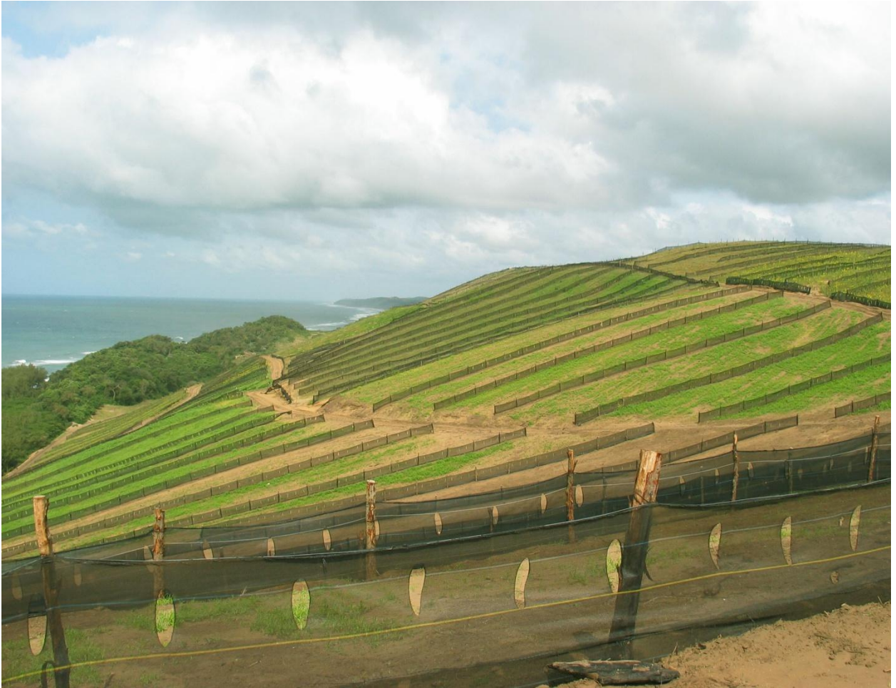
Plate 7-1. Post-mining dunes are re-shaped and then previously stored topsoil is placed on the dune and spread evenly across the site. The erection of shade-netting fences, acts to reduce soil erosion resulting from the action of the wind. Exotic annual herbaceous plants are seeded to further ensure soil stability. The above plate shows a 1 year old site. The photograph was taken by Prof. R.J. van Aarde and is used with permission.
