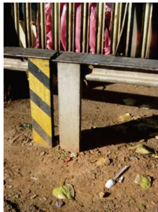
Figures 3.22 and 3.23: The use of old rail lines for street furniture compliments the overall image of the
