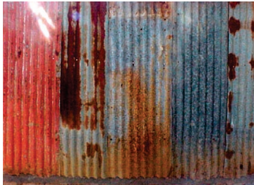
Figure 4.11 Second-hand profiled steel sheeting is used to build houses in both informal and formal settlements. The untreated material ages over time due to harsh climatic conditions, leaving it stained. The dialogue of this material is to be continued on the skin cladding system of the overnight accommodation building
