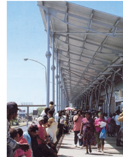
Figure 3.6 The roof structure helps define the public passage. The pitch of the roof opens this facade, celebrating the functions that align it
