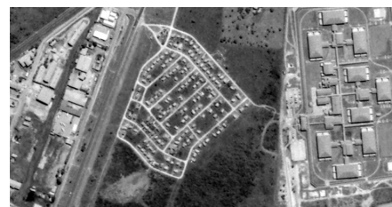
Figure 1.20 Prison housing placed adjacent to N1 Highway
