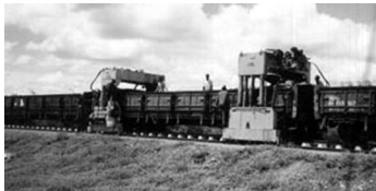
Figure 1.11 Construction of railway line at Beit Bridge
