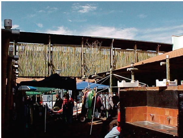
Figure 3.41. View of courtyard walls made of lathes
