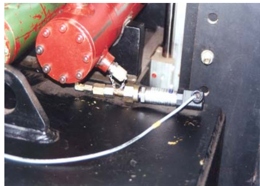
Figure 4-5: 40MPa pressure sensor measuring accumulator pressure
