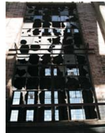
fig 5.22 Power station: derelict
