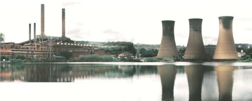
fig 4.1 Northern elevation of site
