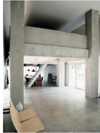
fig 4.14 Water tower house interior
