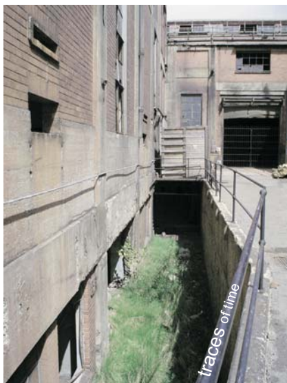
fig 4.2 Derelict power station "A"
