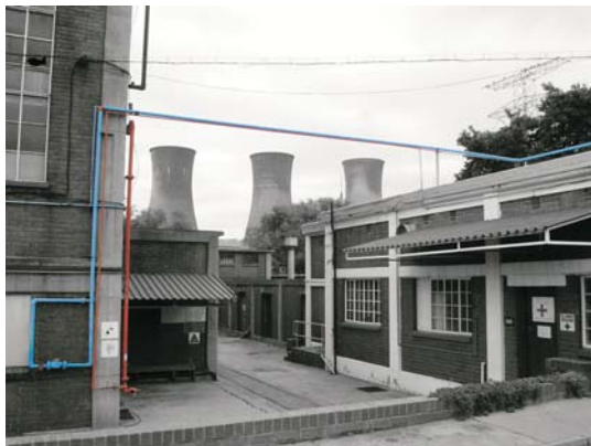
fig 4.16 Abandoned power station
