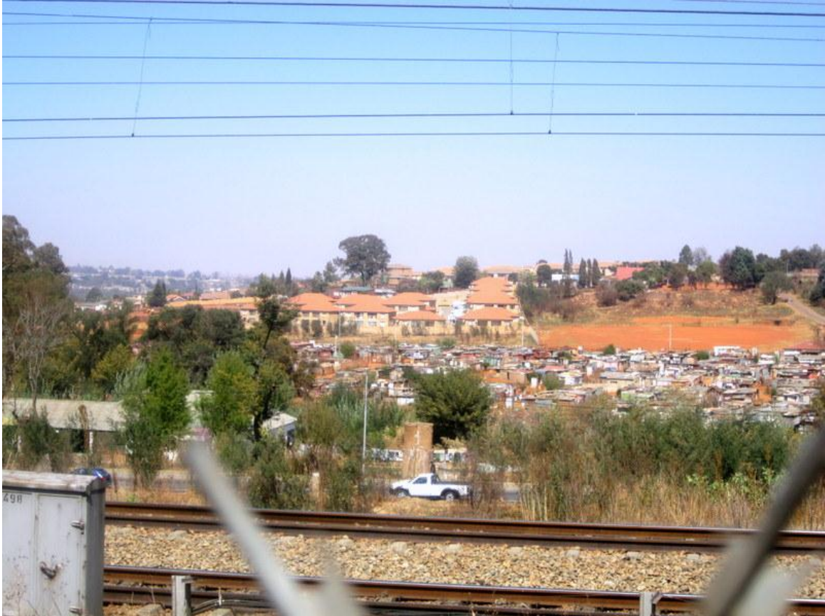
Shacks within the upmarket Princess Crossing in Roodepoort
