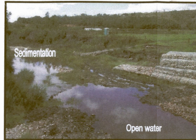
Figure 137: Sedimentation downstream of the gabion structure at site 5.
