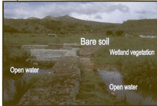
Figure 136: Gabion structure at site 5 (Hudsonvale) of the Kromme River Wetland.
