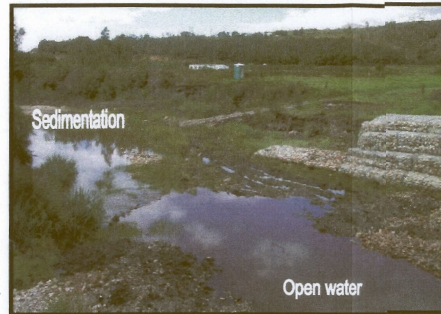
Figure 110: Sedimentation downstream of the gabion structure at site 5.
