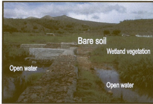
Figure 109: Gabion structure at site 5 (Hudsonvale) of the Kromme River Wetland.
